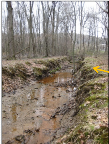
Downstream Commercial Park
